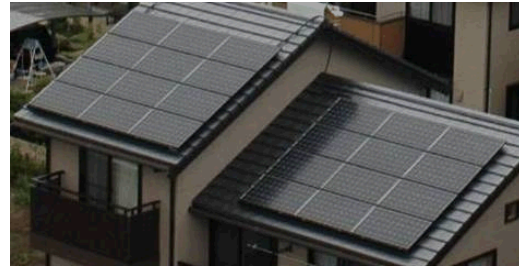
Figure 2: Photo of analyzed PV system
