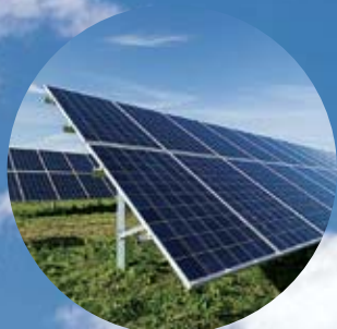
Photovoltaic power generation 太陽光発電
