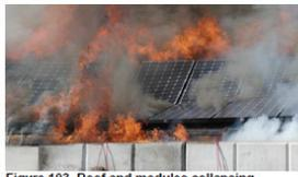
Figure 103 Roof and modules collapsing
