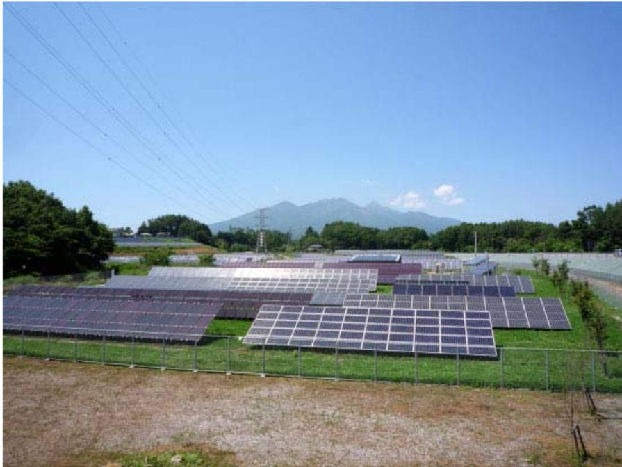
**Figure 1.** The mega-solar system installed in Hokuto, Yamanashi, Japan. About 30 types of PV systems have been installed.
