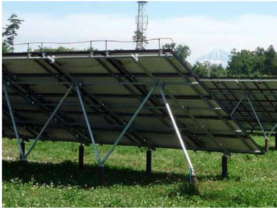
Figure 3 Simplified array structures installed at the Hokuto city
