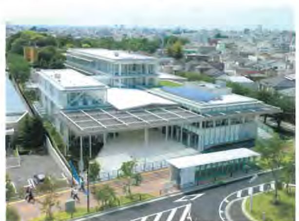
Fig. 5 “Tokyo Tech Front” built in May 2009 at the main gate of Tokyo Institute of Technology. The equipments have been installed here.
