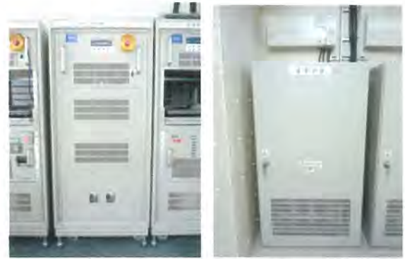
Fig.7 Power router (left) and Power conditioner and Battery (right)
