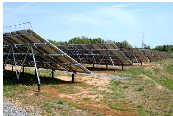
Figure 5: Simplified array structures installed in Hokuto city
