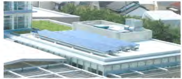
Fig.6 10 kW PV system installed on rooftop of Tokyo Tech Front
