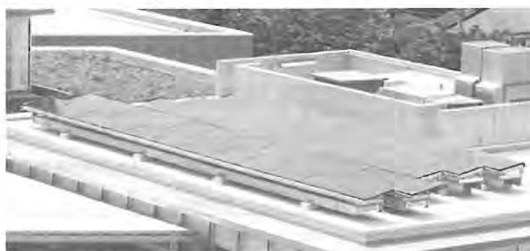
Fig.5 10 kW PV system installed on rooftop of Tokyo Tech Front
