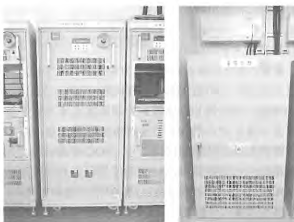
Fig.6 Power router (left) and Power conditioner and Battery (right)
