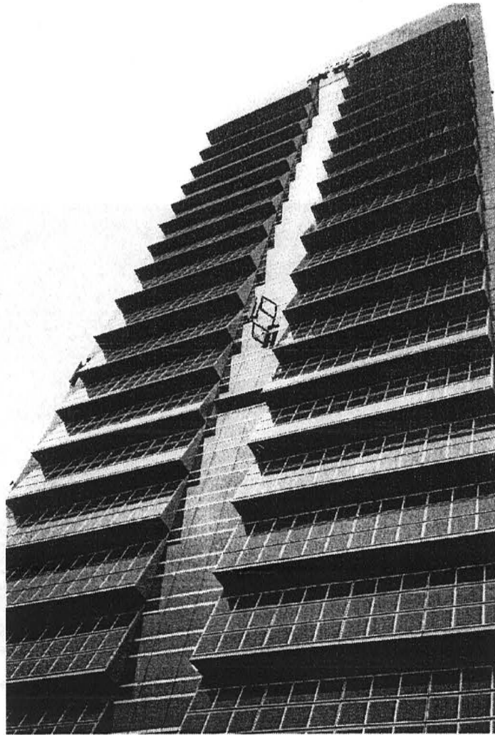
Fig.7 20-storied Kyocera HQ, Kyoto PV: 214kW with gas engine cogeneration distributed inverters; self-shading
