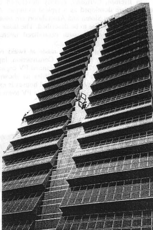
Fig.7 20-storied Kyocera HQ, Kyoto PV: 214kW with gas engine cogeneration distributed inverters; self-shading
